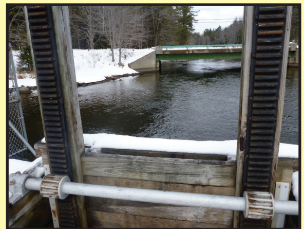
Wing's Mills Dam opened 5 feet for drawdown.
